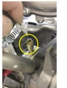
2d-1 Install new fuel line from regulator onto carburetor adaptor inlet after installing correct fuel orifice.
